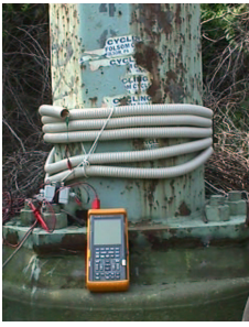
Measuring AC leakage currents in transmission line towers.
