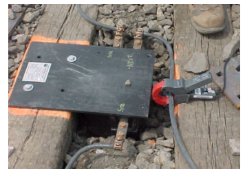
EMA has evaluated the effectiveness of impedance bonds for induction mitigation.
