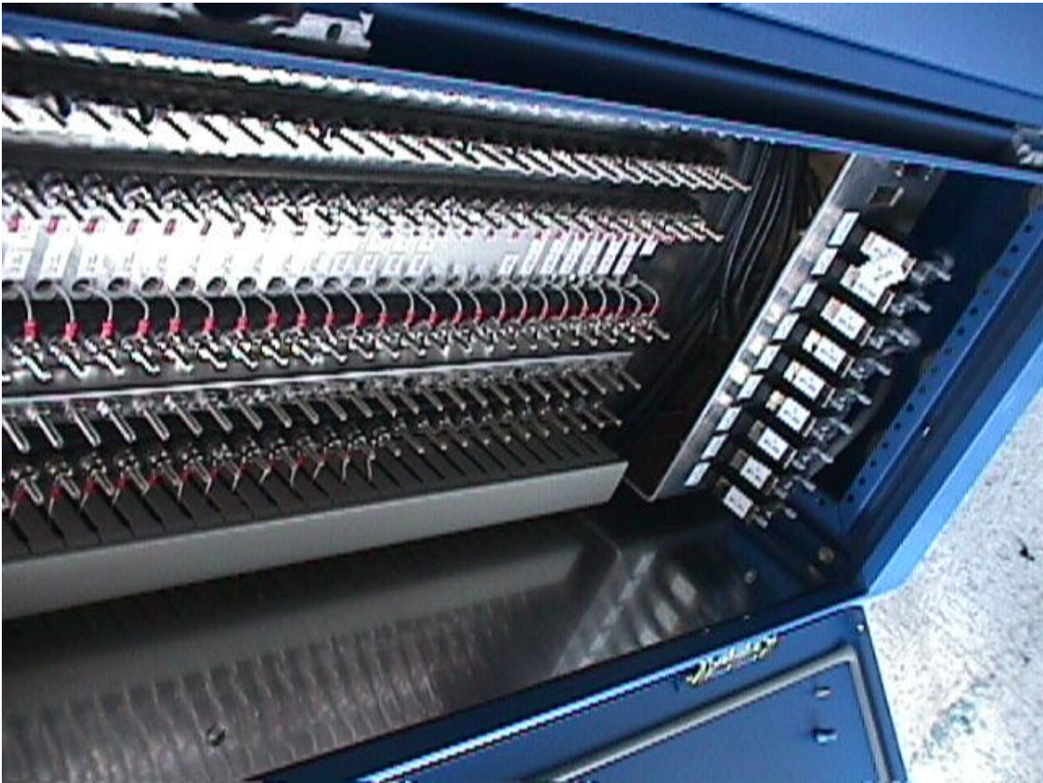
An Example of a Faraday Cage Implementation for Hump Yard PCS Protection
