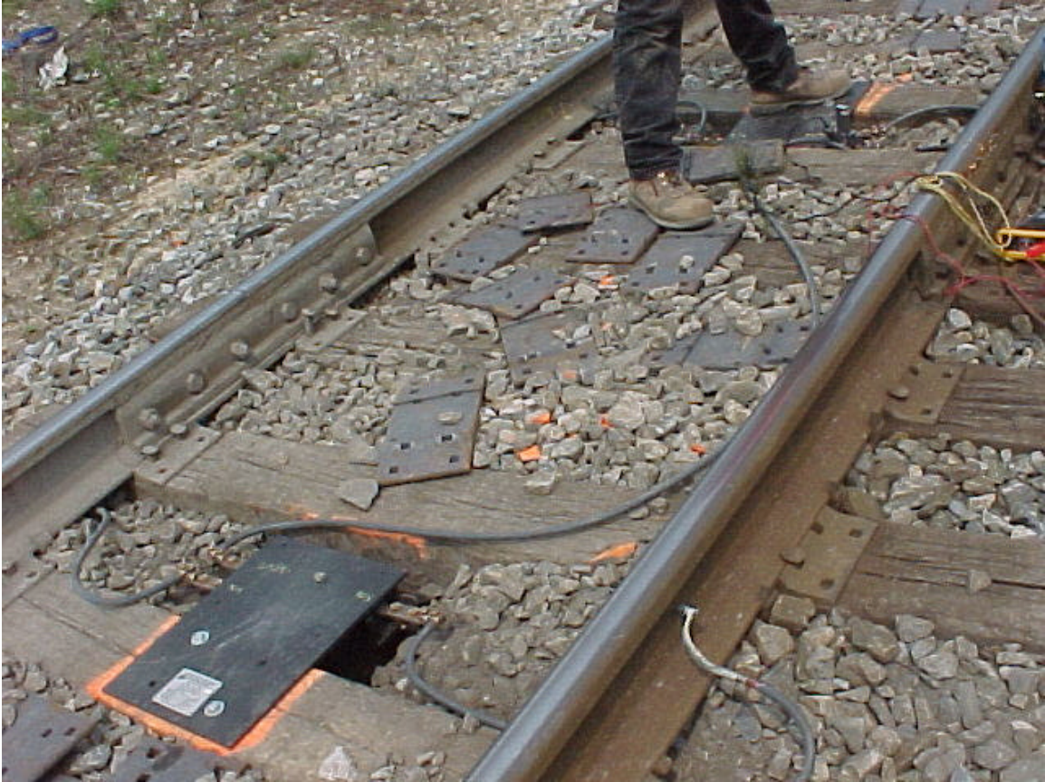
Implementation of impedance bond induction mitigation
